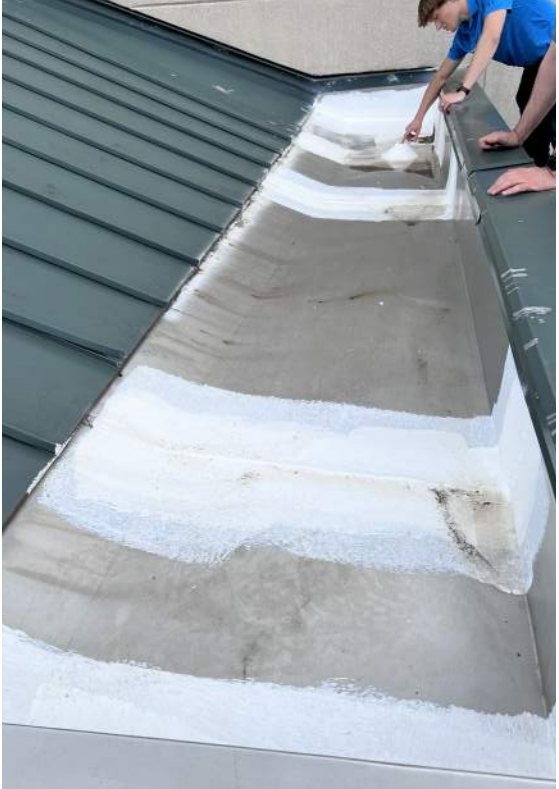
Leaking roof gutter
