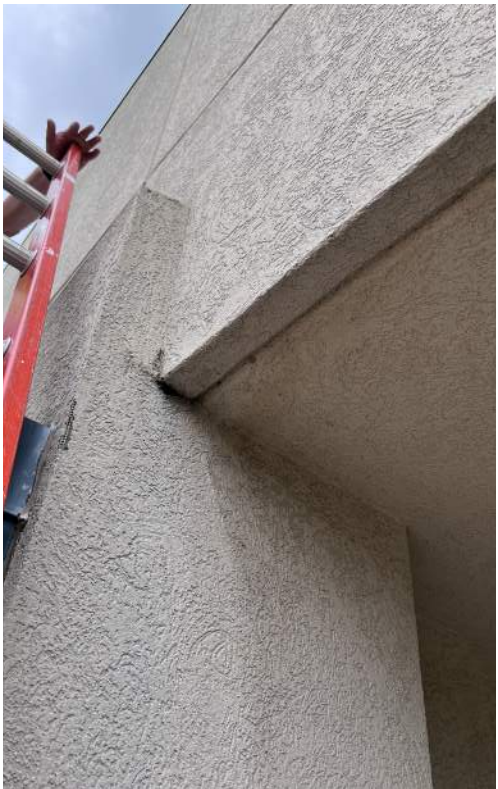
Damaged EIFS cladding
