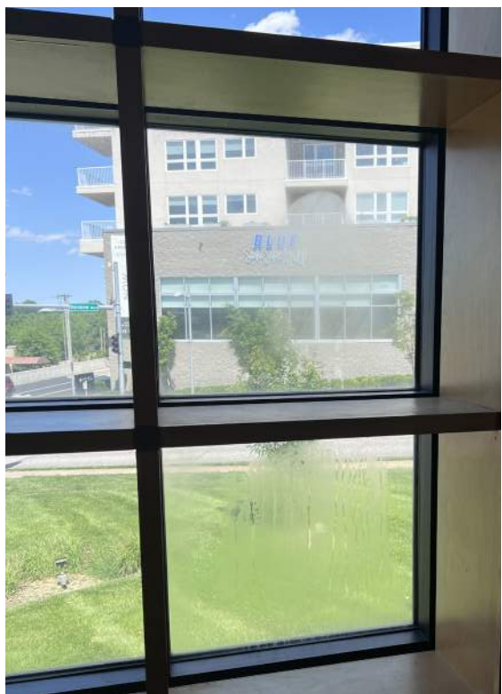
Failing glazing units
