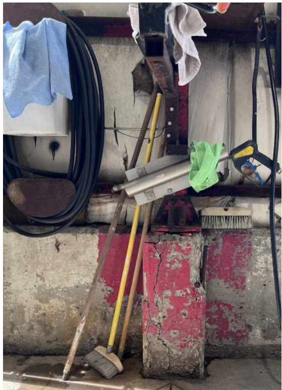
Damaged concrete column foundations
