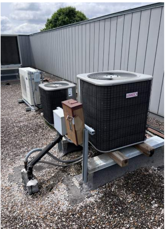
Mechanical units on original ballasted roof
