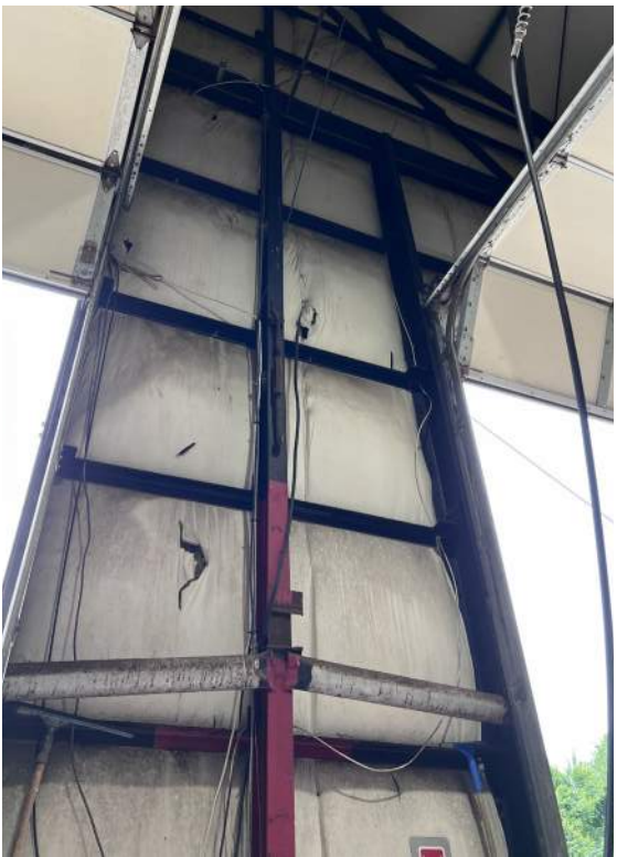
Damaged insulation on wall panels
