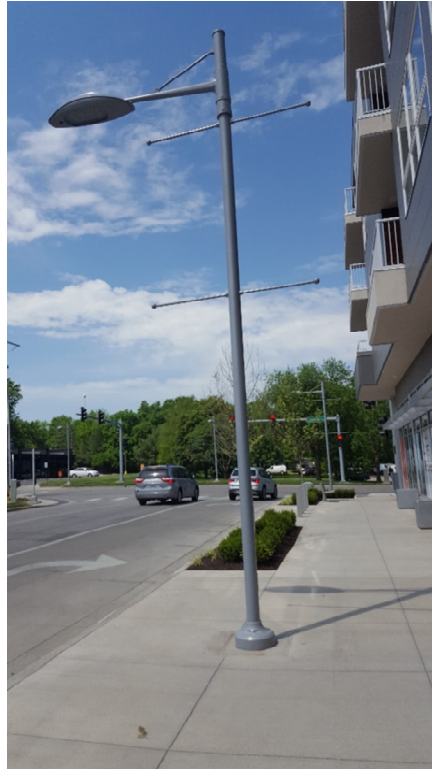
Image 4: Decorative LED Fixture on Metal Pole
